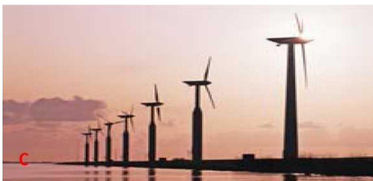
Figure 1: Some important applications of the Law of Hydrodynamic Pressure. The pressure plays a key role in power plants (A), piping an plumbing system (B) and wind turbines (C).
